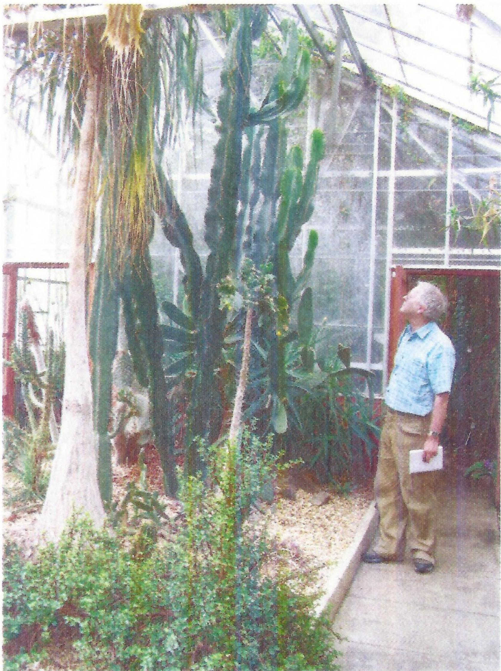
The central section in good condition
